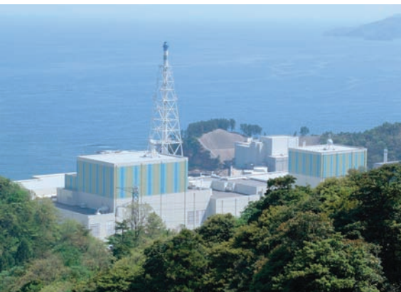
Shimane nuclear power plant, Japan
