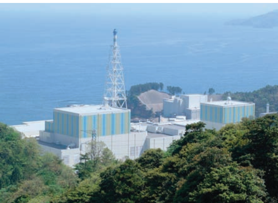
Shimane nuclear power plant, Japan
